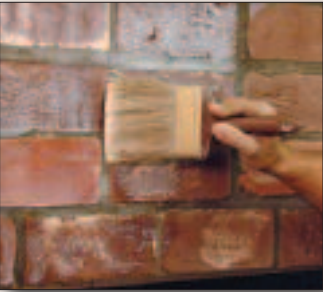
For best results always use a bonding agent when installing Veneerstone directly over concrete, masonry, stucco, brick and block.
