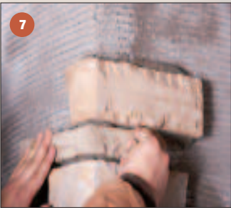
Install corner stones first.
